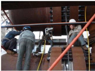
● 炼油厂压力容器螺栓预紧
