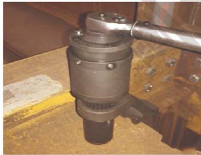
● 钢结构螺栓预紧
