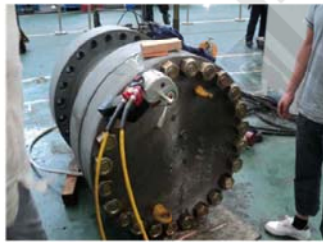
● 钢厂高压管道法兰盘螺栓预紧
