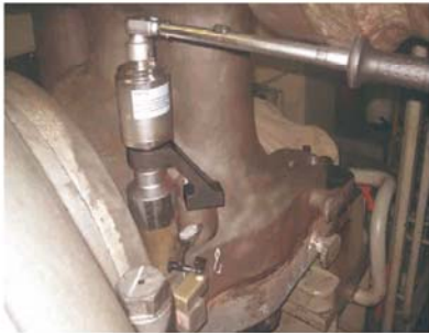
● 大型压力容器螺栓预紧
