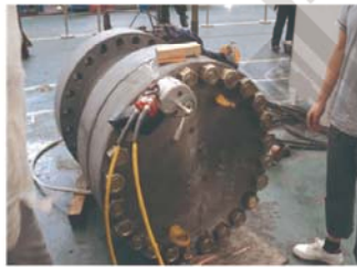
● 钢厂高压管道法兰盘螺栓预紧
