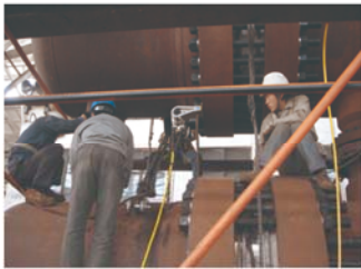
● 炼油厂压力容器螺栓预紧
