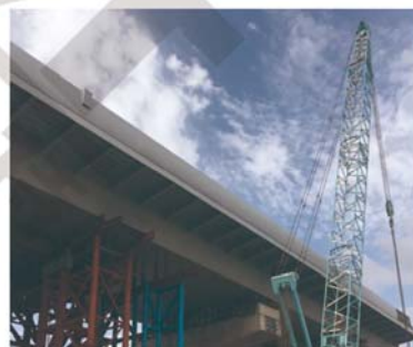
● 钢箱梁跨高速公路同步顶推
