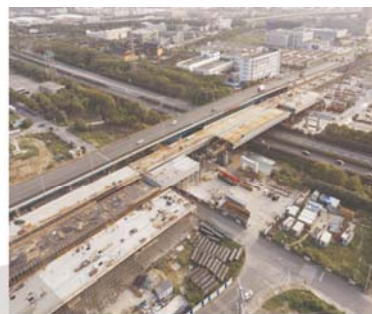
● 钢箱梁跨高速公路同步顶推
