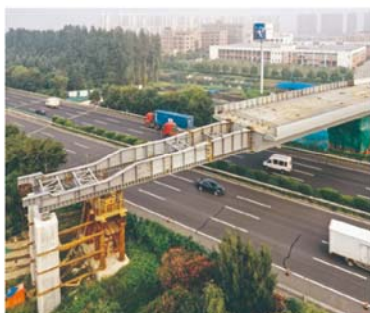
● 钢箱梁跨高速公路同步顶推
