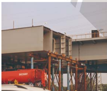
● 钢箱梁跨高速公路同步顶推
