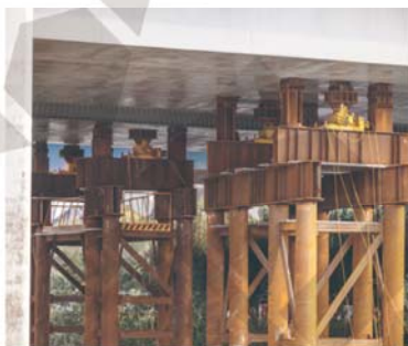
● 钢箱梁跨高速公路同步顶推
