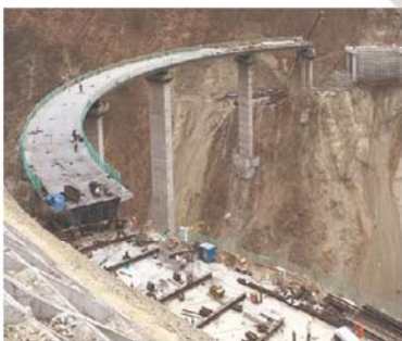
● 钢箱梁匝道同步顶推
