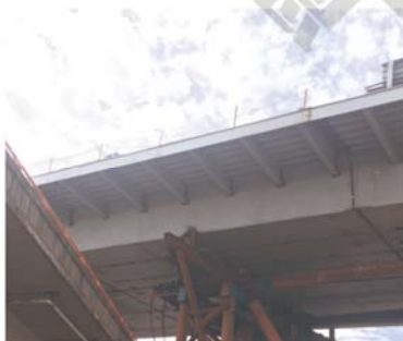
● 钢箱梁跨高速公路同步顶推
